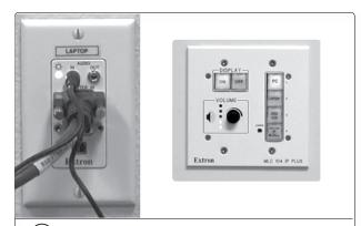
(3b) Connect and turn on the input devices, and turn on the display at the MLC
