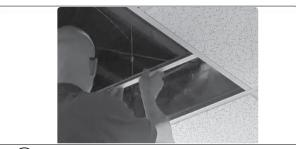
(2a) Place the T-rails on the T-frame
