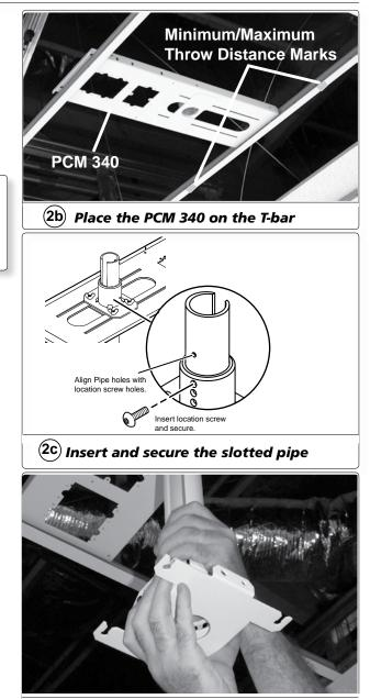
(2d) Screw the adjuster plate onto the base
