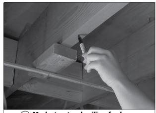
5a Mark structural ceiling for lag eye bolt installation
